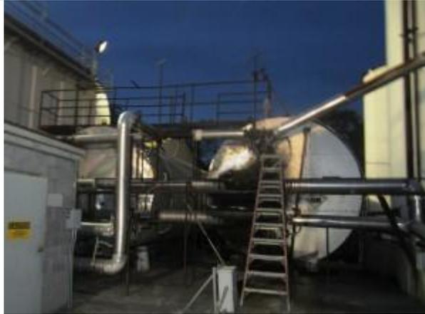
*The asphalt cement came to Virginia Paving's tanks already blended with the SonneWarmix and ready to mix for the Balls Hill Road project.*
